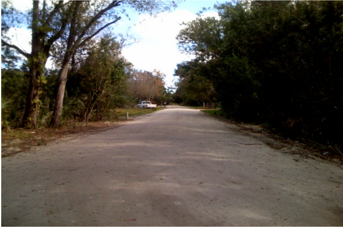
County Road After Work
