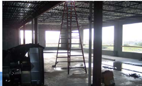
2nd Floor - Southeast corner
